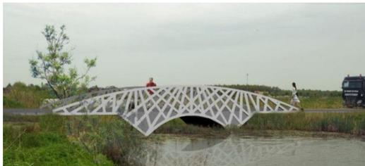
3D printing bridges isn't new per se. Earlier this year, we reported on the first 3D printed pedestrian bridge in the world, located in Madrid, and in the Netherlands there is a 3D printed metal bridge. The difference, however, between these bridges and the new ones is the material (metal versus reinforced concrete) and the size (pedestrian versus bicycle and car bridge). 3D printing concrete has several advantages over
