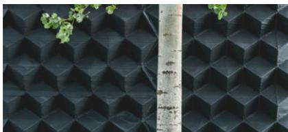
Optimising the construction process and be circular are two important themes currently in the construction industry. Jumping aboard this ship, De Meeuw, a Dutch specialist company in flexible and circular construction, and Actual, the 3D label of the Amsterdam architect firm DUS Architects, are collaborating in a project to create 3D façades made from recycled waste. With 3D printing, they
